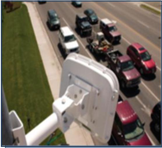
The Department has been testing the SmartSensor over the last month at the intersection of Columbus Parkway and Ascot Parkway. The radar detector is mounted on a signal pole and is currently being used to alert the traffic control box of vehicles wishing to turn left from northbound Columbus Parkway onto westbound Ascot Parkway.
