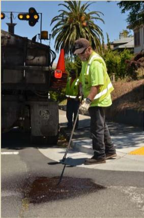
This project was one of the City's infrastructure investments using Measure B funds. The streets that were slurry sealed had small potholes repaired and large cracks filled, before a tarry emulsion was applied to the entire street to minimize water intrusion to the road bed. Without the slurry seal, the potholes and pavement would ultimately fail. For a list of streets that were scheduled to be sealed [click here](#).
