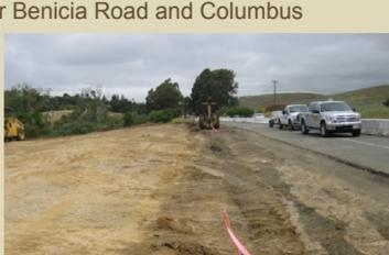
The SWMP is being built to accommodate the increased rainfall runoff caused by building the new homes. This holding area will tie into an existing 48-inch storm water drain. A maintenance road is also being built for easy access to the new water detention area as well as the existing one. The sidewalks and widened road will extend approximately 300 feet up Benicia Road from Columbus Parkway, and 500 feet north on Columbus Parkway. View the planning design scheme [here](#).
